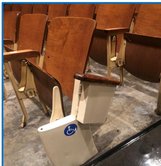
Exhibit B.8: Modified auditorium seating and arm rest
