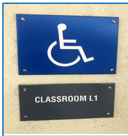
Exhibit B.12: Installed visual and tactile signages
