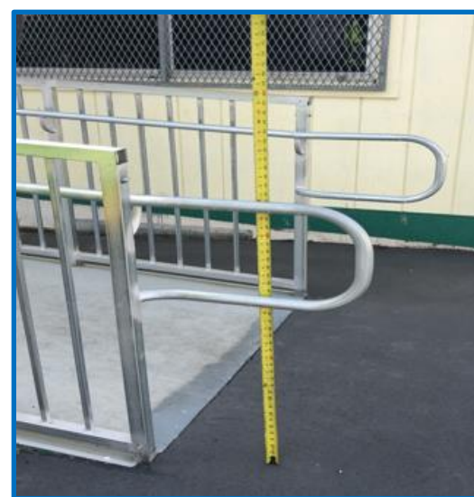
Exhibit B.3: Measured height of handrails
