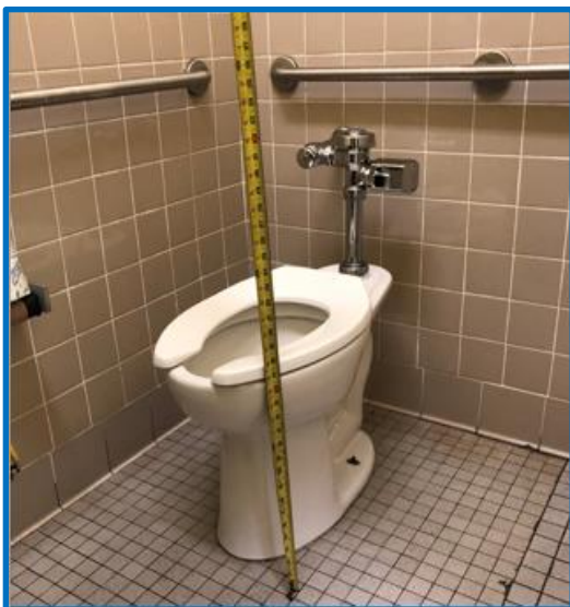
Exhibit B.4: Measured height of toilet seat
